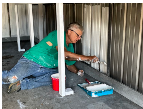
Kevin Wilson painting the inside of the Loan Closet storage building that was damaged last year by a fire. Thank you Kevin!
