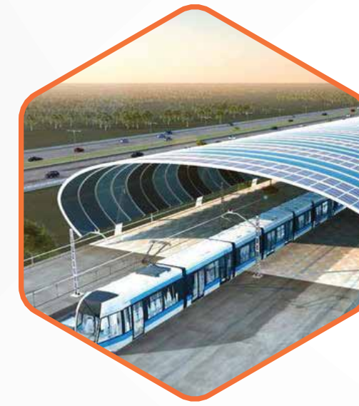
Ahmedabad - Dholera Metro
