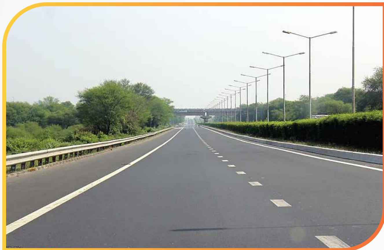
Pipli - Vataman - Baroda Six Lane Highway 500 MTR
