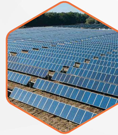
World's Biggest 5000 MW Solar Park in 110 Sq. Km.
