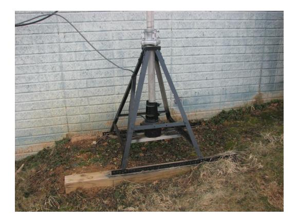
Here is an example of a post mounted push-up mast with a hex beam using a thrust bearing for more support:
