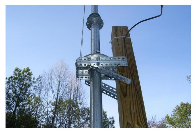
Another example, this time of the rotor at the bottom of a postmounted mast.
