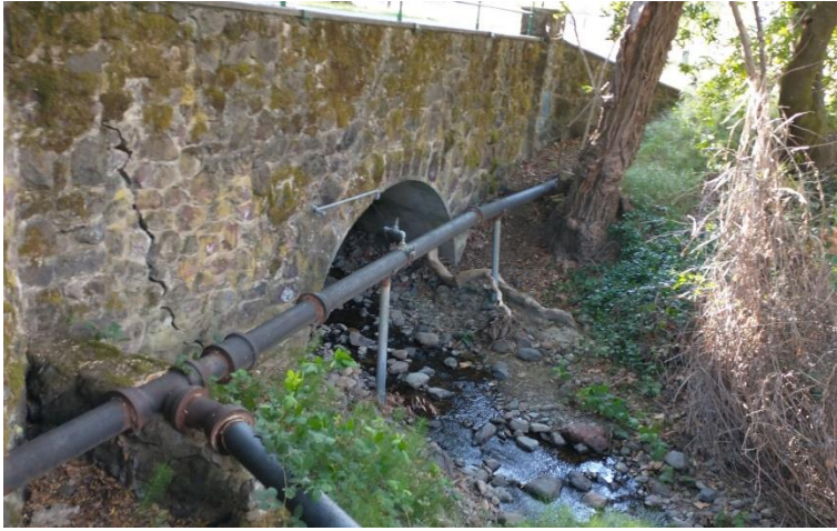
Figure 10 and 11. Two examples of pipes crossing Mill Creek, two of many such crossings. Project proposes to re-construct a new grid of water/sewer pipes, but the Project does not specify whether it will leave these lines in place (abandon them) or remove them as part of demolition. We think abandoned pipes should be removed, in coordination with the appropriate agencies and protections.
