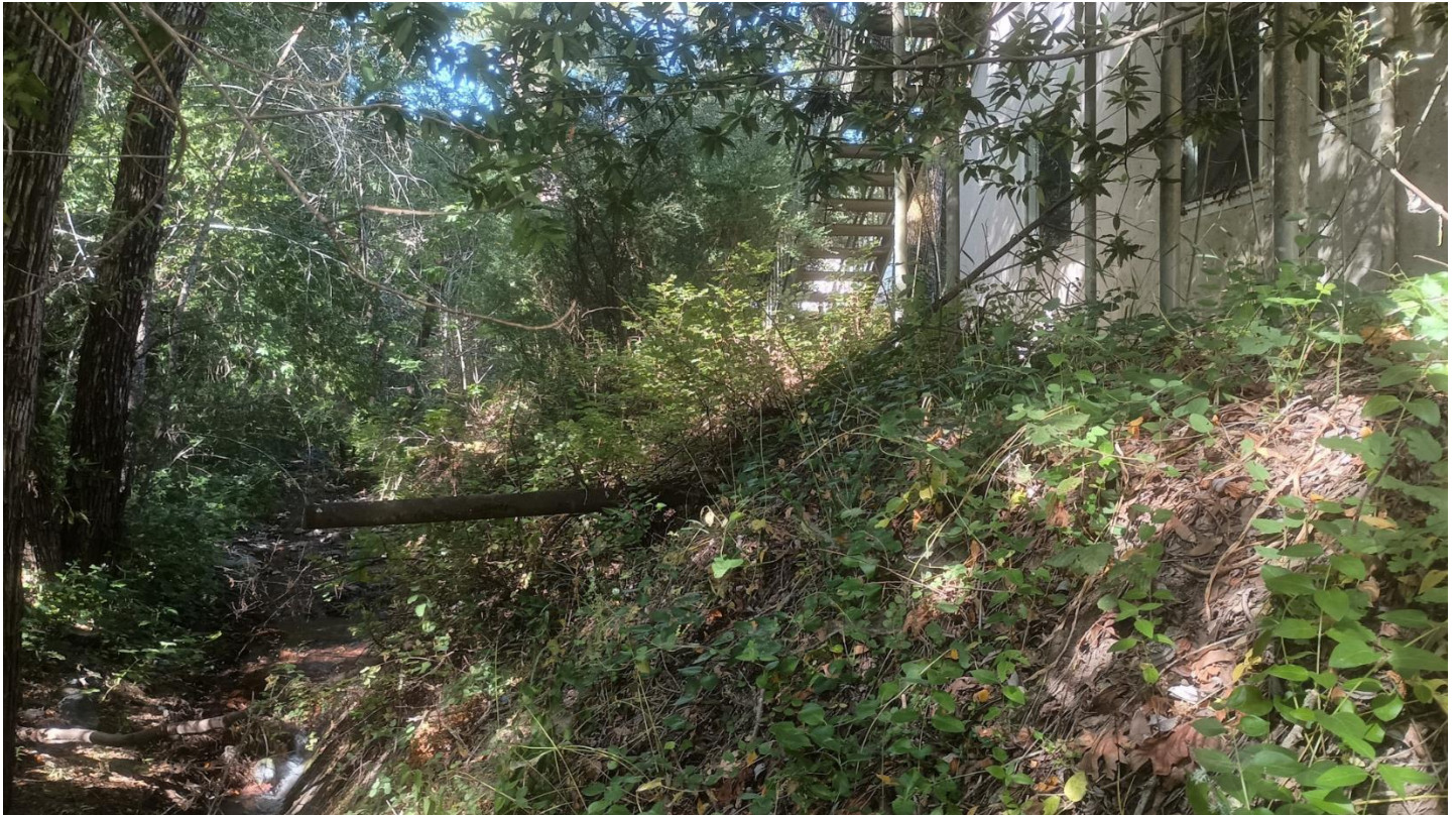
Figure 9. Example of existing infrastructure (slated for demolition) that is congruent with the top-of-bank of Mill Creek. Mill Creek is visible in the lower left, as is a storm drain entering the creek. There are about 6000 linear feet where demolition is planned within a few feet of the top of bank. Standard construction stormwater measures won't suffice.
