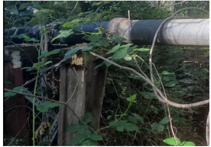
Figure 10 and 11. Two examples of pipes crossing Mill Creek, two of many such crossings. Project proposes to re-construct a new grid of water/sewer pipes, but the Project does not specify whether it will leave these lines in place (abandon them) or remove them as part of demolition. We think abandoned pipes should be removed, in coordination with the appropriate agencies and protections.
