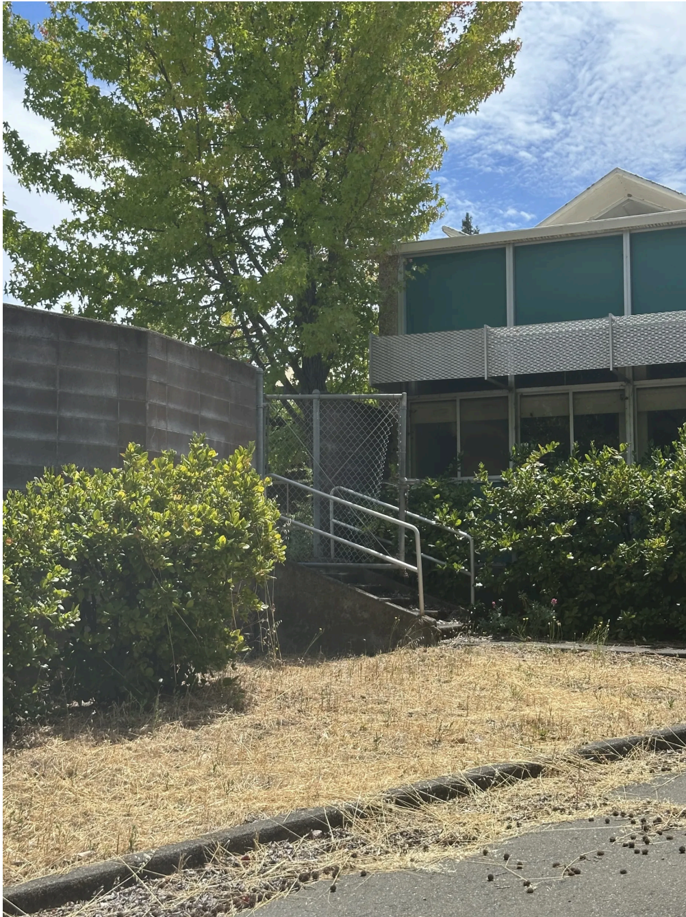
Gates around the Nelson building have been left open. (The Sonoma Index-Tribune)
