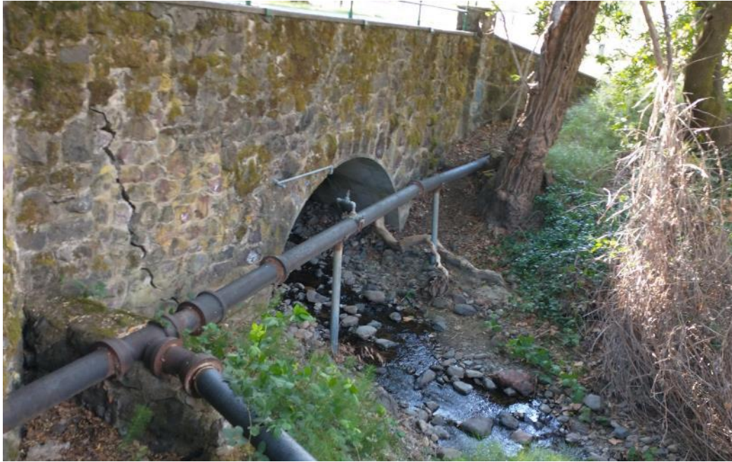
Figure 6. Pipes crossing Mill Creek at the existing bridge, one of many such crossings. Although the Project proposes to abandon existing lines and re-construct a new grid of water/sewer pipes, the
