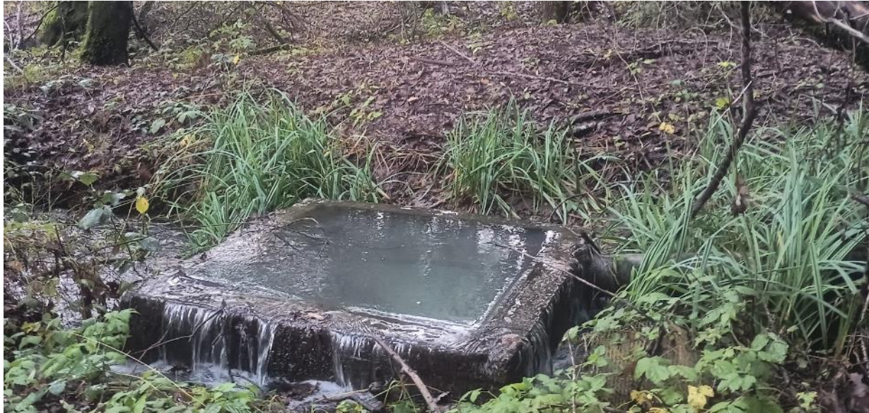
Figure 4. Current condition of the main collection box at Roulette Springs, located on former SDC land now owned by State Parks. Infrastructure is more than leaking; it is non-functional. Water is spilling onto the forest floor. The spring complex creates in-situ wetlands and provides the base flow for Asbury Creek during summer months. The spring is also a critical component of the Project's proposed water supply, providing a large fraction of total water supply, especially during summer months and multi-year drought periods. We feel the EIR must analyze potential impacts of water system development.
