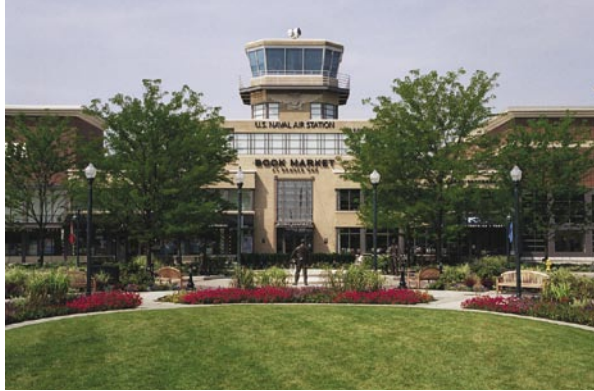
The former control tower was converted into a bookstore at Glenview Naval Air Station.
