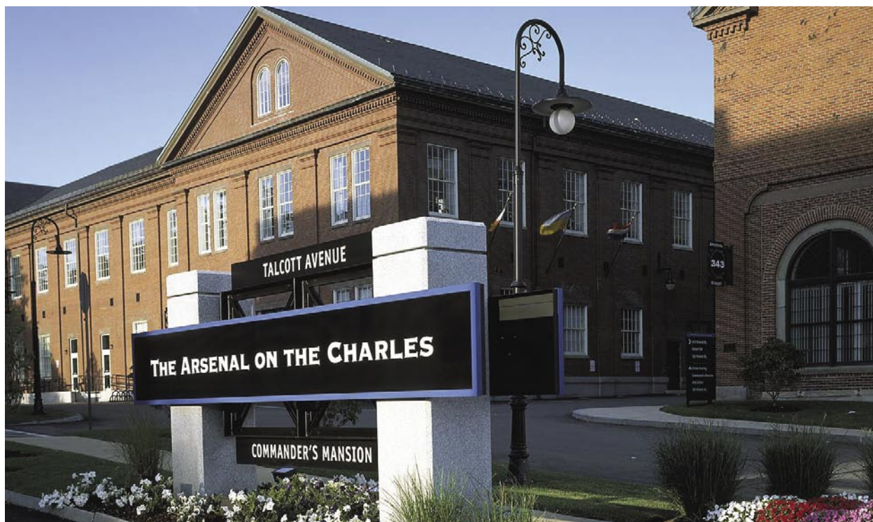
The historic brick buildings of Watertown Arsenal outside of Boston, Massachusetts.
