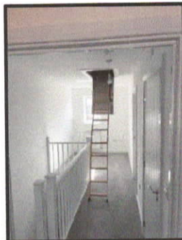
Fitted ladders to boarded lofts
