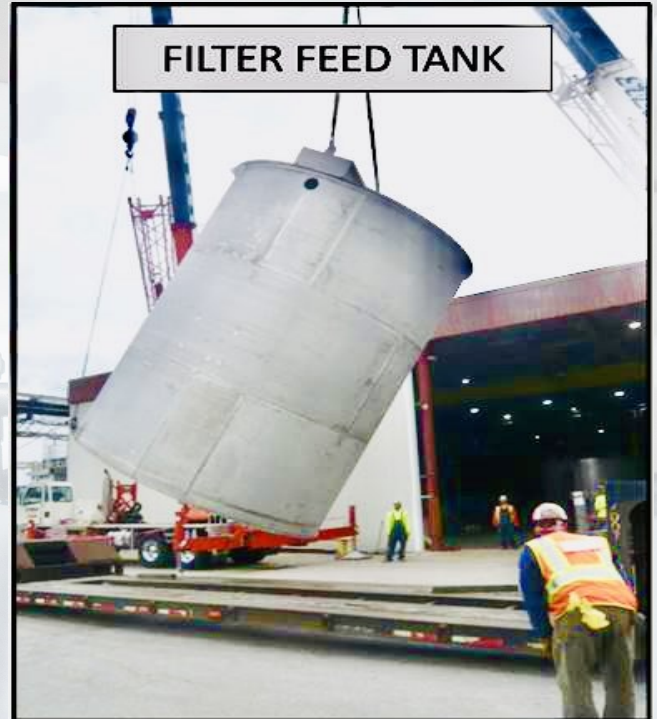
16,000 Gallons Capacity Storage Tank
