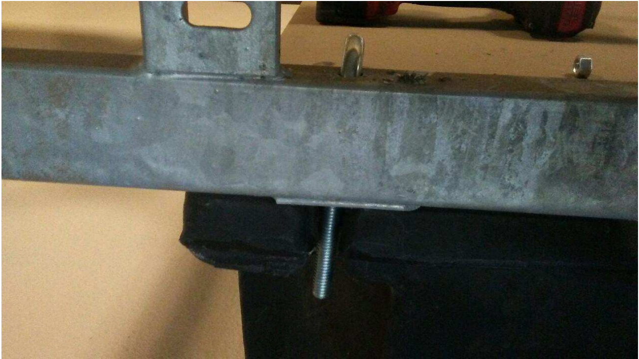
Properly connected J bolt to float ready for large SS washer, flat washer, lock washer, and nut
