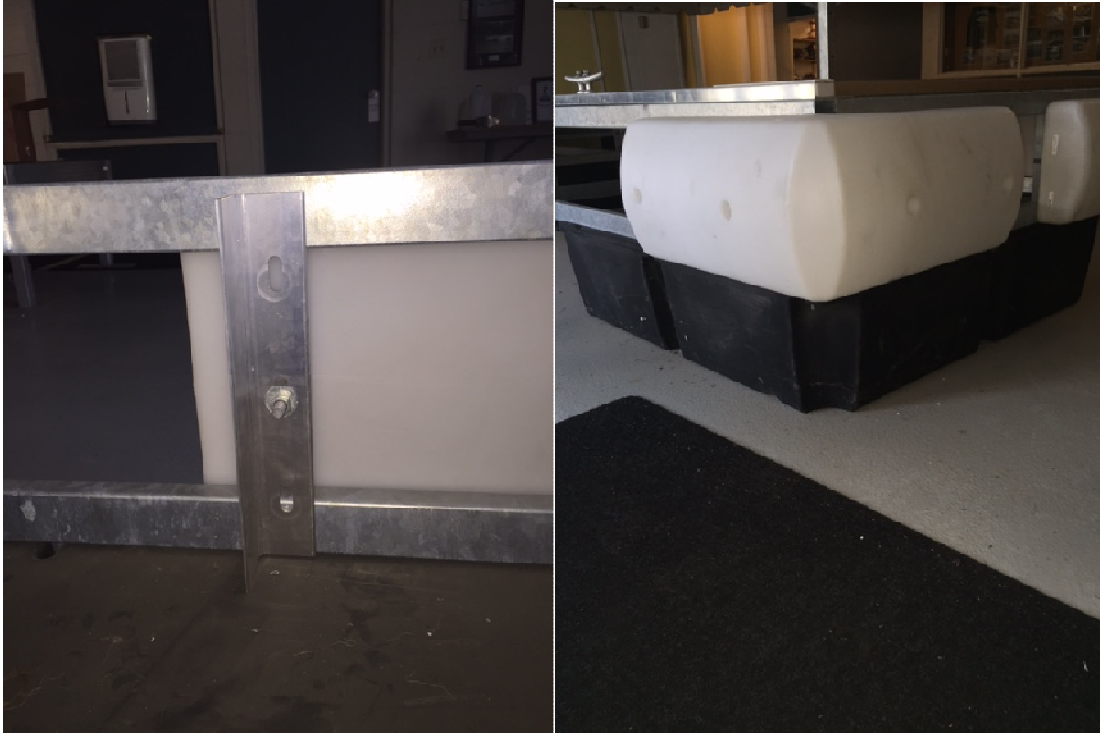
Mounting bracket and bumper installed (corner mount shown)
