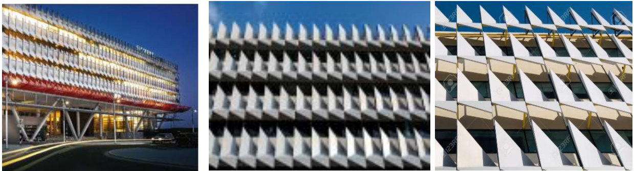
Fig-12 Siemens regional headquarters -Foster and Partners Consultants started 2008
