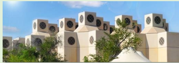
Fig-6 The Qatar university ventilation towers
