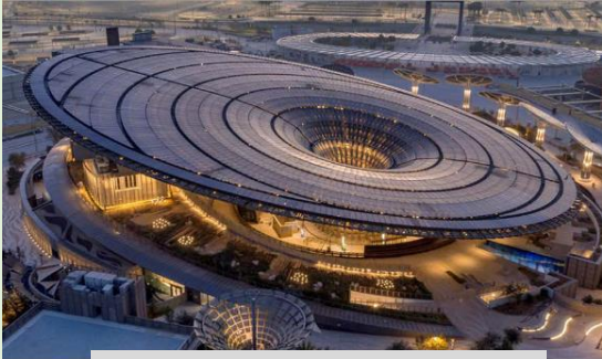
2021 Net Zero Building Project of the Year Terra – The Sustainability Pavilion Expo 2020 Dubai
