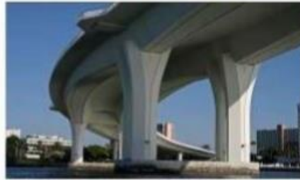
Green concrete bridge
