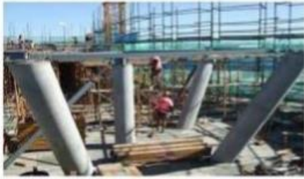
Green concrete columns
