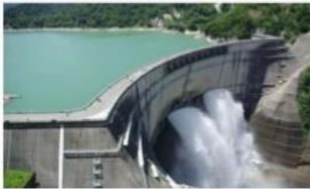
Green concrete dam
