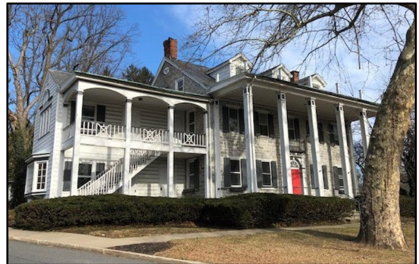
OASIS Community Center
