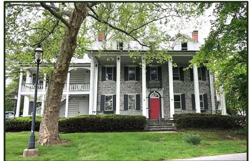
OASIS Community Center
