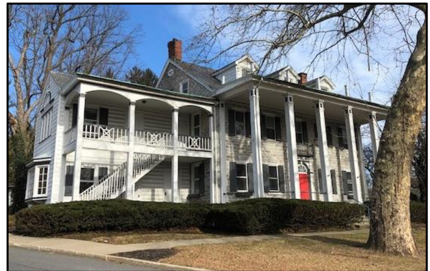
OASIS Community Center
