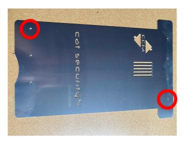
Step 2 - Once the Cat Security<sup>TM</sup> shield is stable, proceed to drill out the inner holes for the rivets. Install the rivets using the 1/2° rivet gun.
