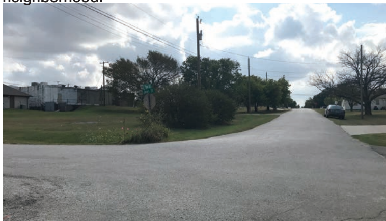
Existing south view of Pine Street at the corner of Jearl Street
