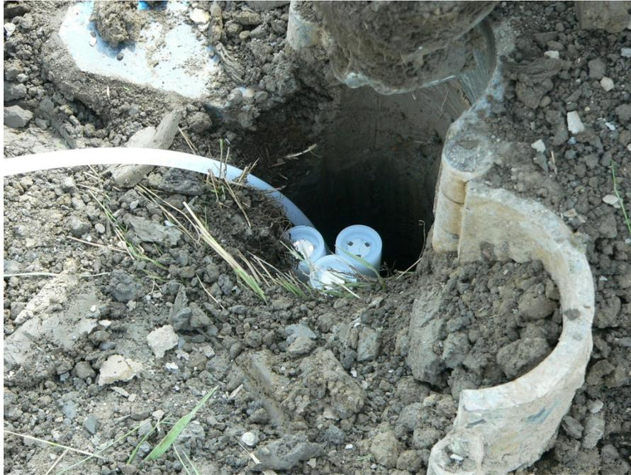
*Figure 13. 20-ft. EGRP nest installed 4-inches below grade.*
