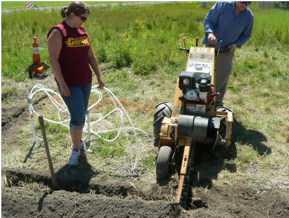
*Figure 19. Self-propelled trenching machine cutting the trench for the infiltration pool walls.*
