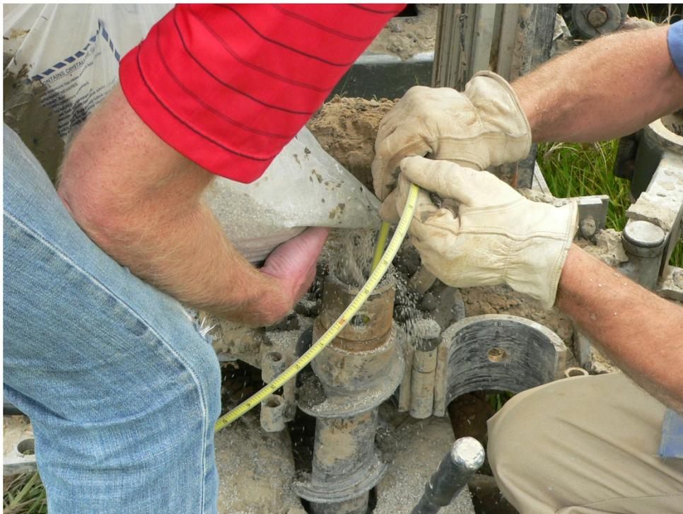
Figure 10a. Sand packing one of the monitoring wells (sealed 3/4" riser tube is within the hollow-stem auger about 4 inches below the top of the flight).
