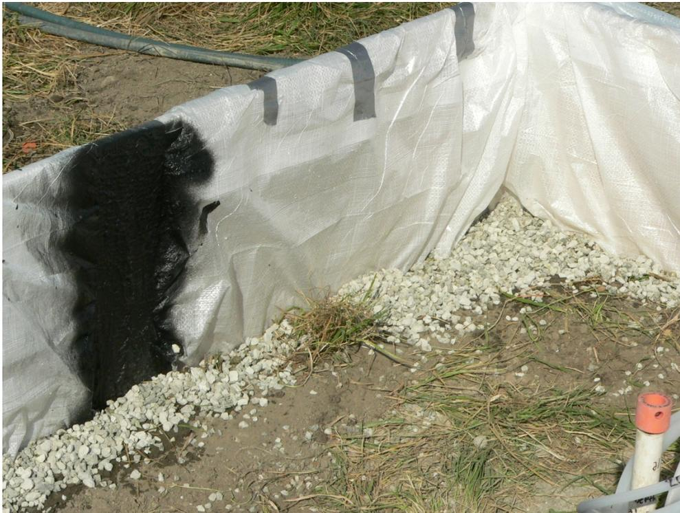
*Figure 22. The inside trenches were filled with bentonite, which was thoroughly hydrated before filling the pool.*
