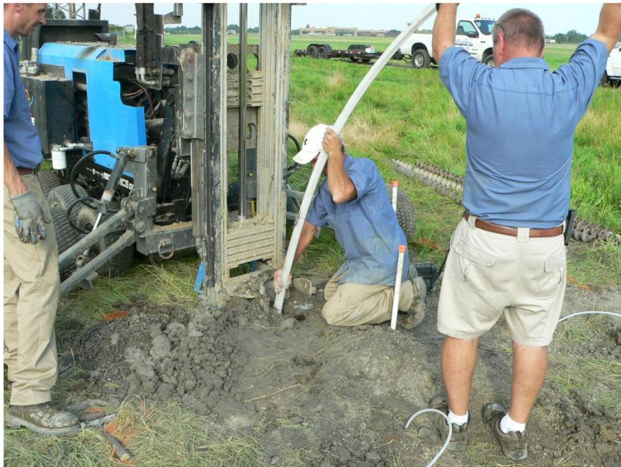
*Figure 14. 40-ft. EGRP nest being installed in an open bore hole that had been drilled with a solid-stem auger.*
