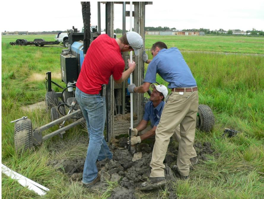
*Figure 8. SME installing a ¾" MW through Heritage's hollow-stem auger.*
