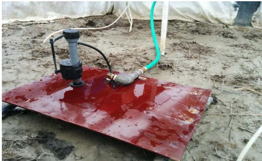
*Figure 25. Custom float valve installed within the infiltration basin. To avoid scouring the bottom of the basin, the valve discharge is dispersed across the metal plate.*
