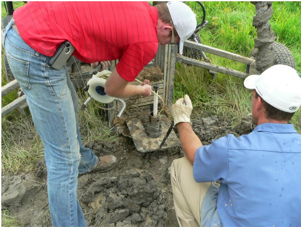
*Figure 10b. Checking the depth of the top of the sand pack prior to grouting the MW.*
