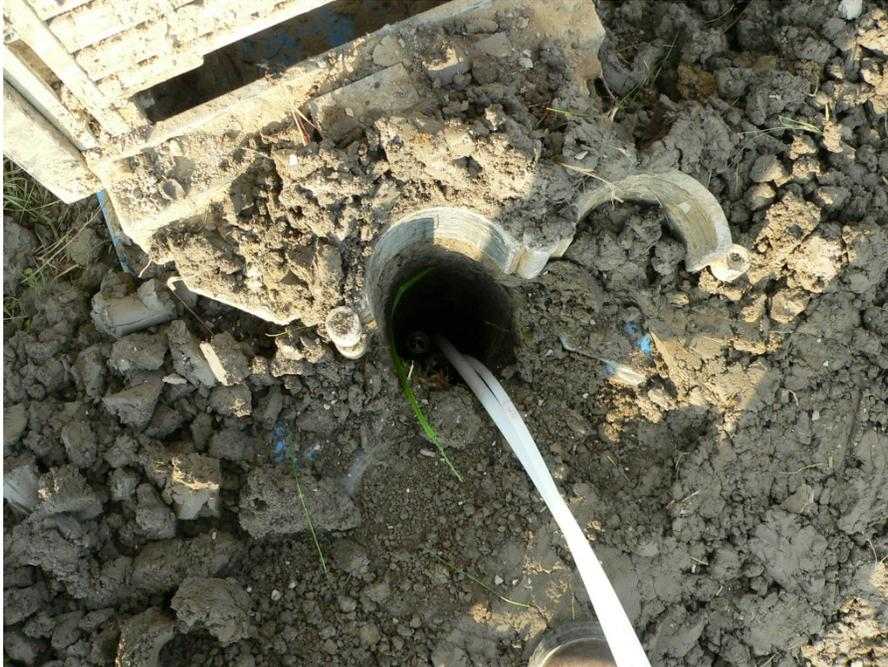
Figure 15. 40-ft. EGRP nest installed 16 inches below grade
