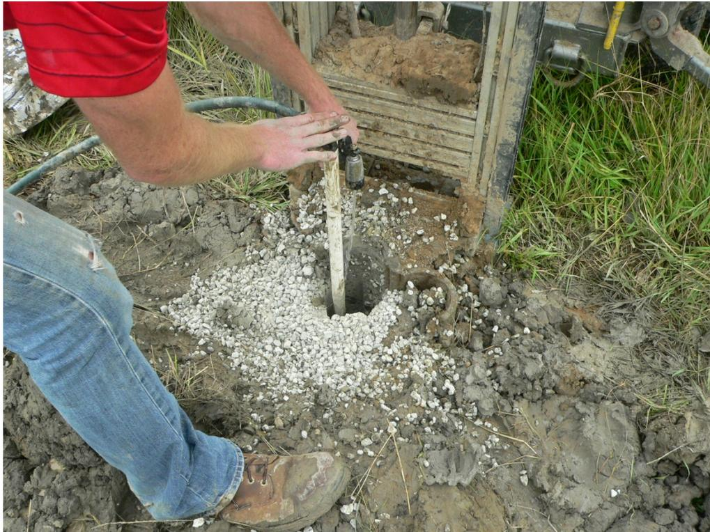
*Figure 11. Grouting one of the MWs using medium bentonite chips (down-hole bentonite being wetted).*
