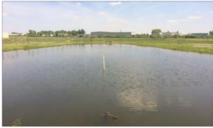
Facing northeast viewing high water level in Forebay. Outlet to Detention Pond is underwater and the staff gauge is in the middle (May 29, 2014).
