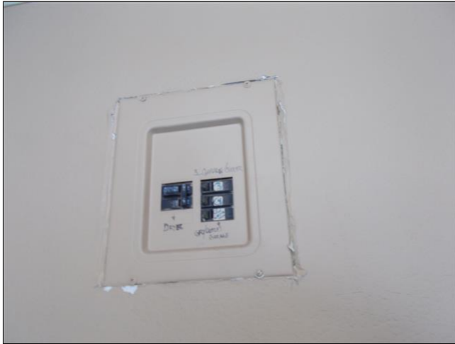
Garage electrical subpanel
