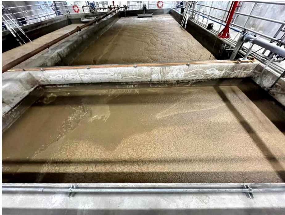
Figure 2: One of the pre-react zones showing floating FOG and some foam accumulating.
