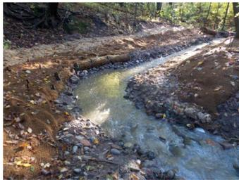
Channel erosion stabilized by rock and coco logs. Bank erosion checked by landscape fabric and seeding.
