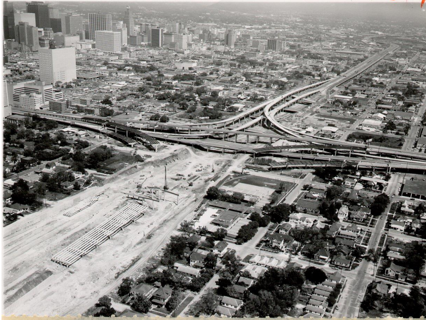
3825 Construction of I.H. 45-U.S. 59 interchange in
