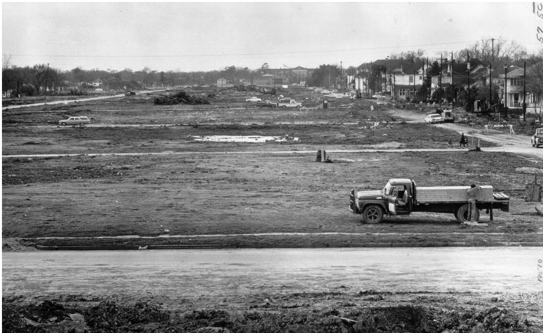
View of Right-of-Way clearing in a residential neighborhood for I-45 where US-59 and SH 288 would merge in Third Ward (1969) 247
