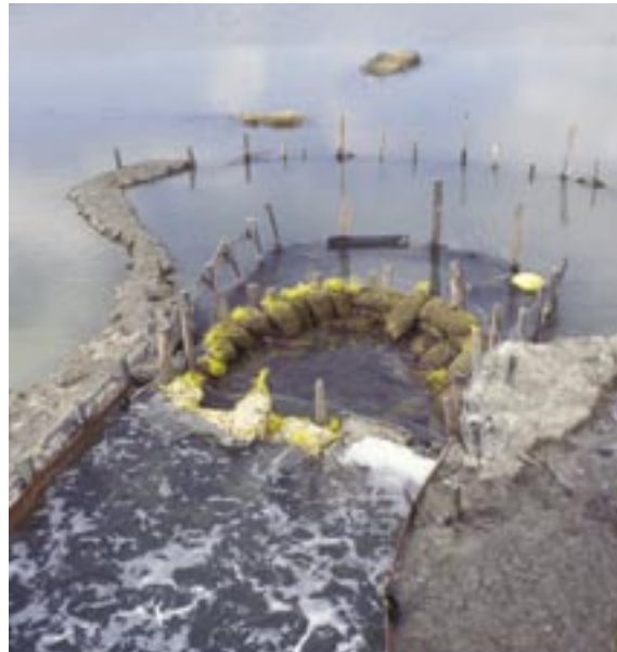
Filtering system made of oyster shells, feathers and pozzolana * at the entrance to mud flats
