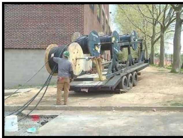
FIGURE 0-11: CABLE PULLED AND GUIDED BY CREWMAN
