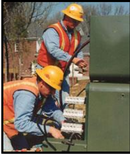
FIGURE O-26: PULLING AND INSPECTING THE CABLE
