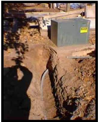
FIGURE 0-1: TRENCH FOR URD CABLE
