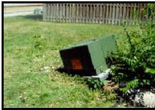
FIGURE 0-2: EXAMPLE OF INCORRECTLY STABILIZED BASE
