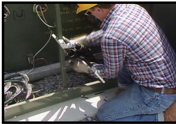
FIGURE 0-8: TYING BACK SECONDARY CABLES AT THE TRANSFORMER
