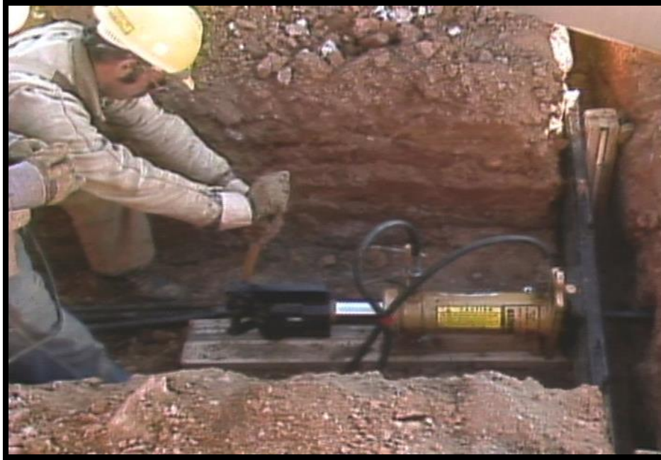
FIGURE O-17: PUSHING A ROD USING HYDRAULIC POWER
