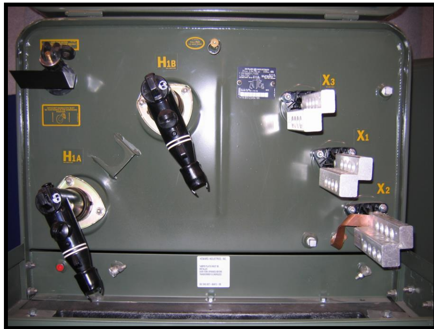
FIGURE 0-5: TRANSFORMER CONNECTIONS
