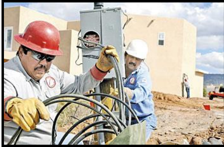
FIGURE 0-25: FEEDING THE CABLE
