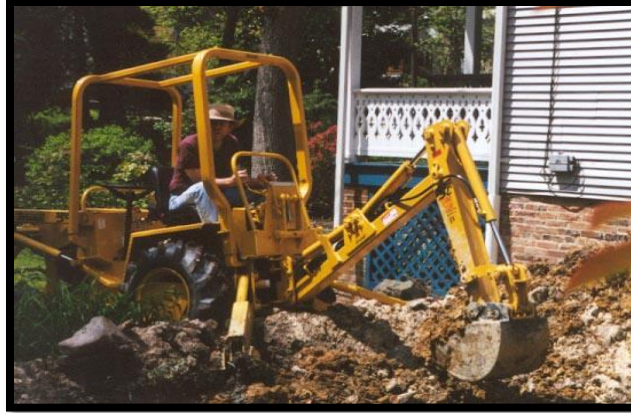
FIGURE 0-8: BACKHOE WORKING IN TIGHT RESIDENTIAL AREA
