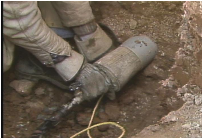
FIGURE 0-22: CONE AND JET LINE GUN IN PLACE
