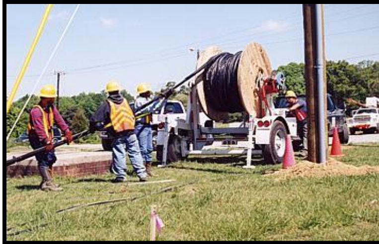
FIGURE 0-10: CABLE PULLED FROM CABLE REEL
