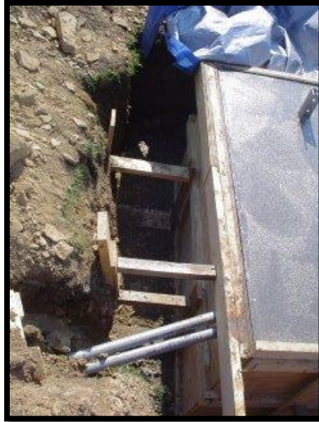
FIGURE 0-4: CONCRETE PAD INSTALLATION
