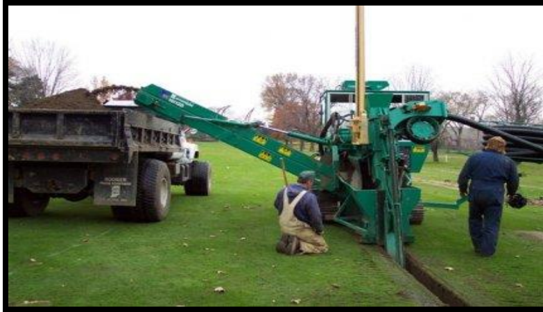
FIGURE O-5: MONITORING THE DEPTH OF A TRENCH
