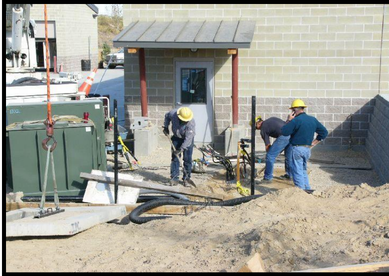
FIGURE 0-5: MOVING THE TRANSFORMER INTO POSITION
