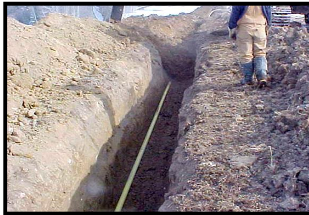
FIGURE O-6: TRENCH READY FOR BACKFILLING
