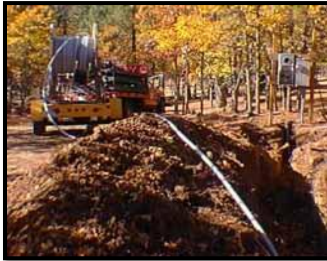
FIGURE 0-12: ROLLING CABLE INTO TRENCH
