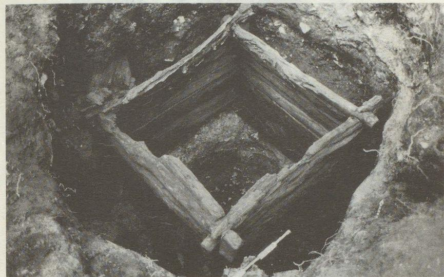
FIG.13 A well with laft construction.
