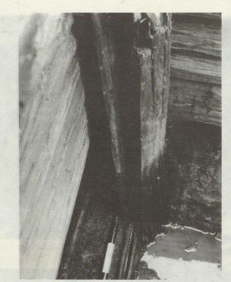
FIG.15 Detail of a corner of a 'sleppveg', together with an earlier lafted well behind it. Note the characteristic grooved post.
