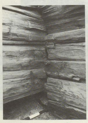
FIG.14 Detail of a corner of a lafted well, (note absence of a beam above scale).
