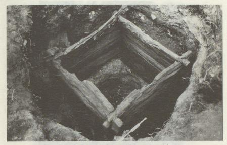
FIG.13 A well with laft construction.
