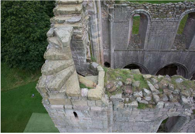
Figure 71 Image taken from a rotary SUA for wall-top inspection. © Skyline Images
