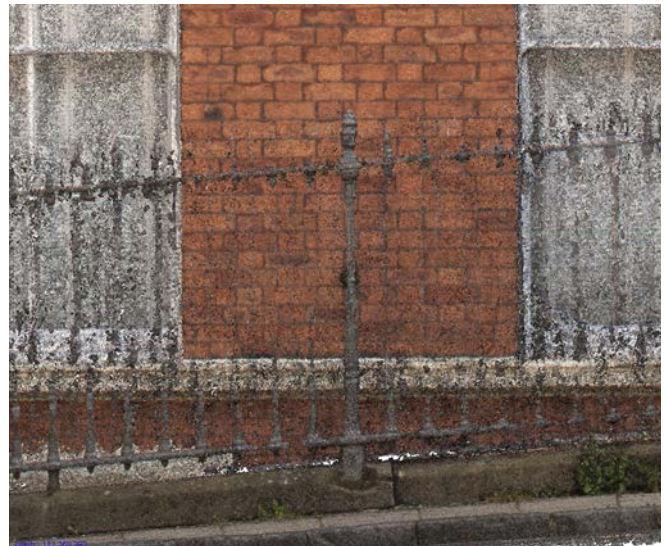
Figure 76 Poor representation of ironwork in an ortho-image from general shots of an elevation.
