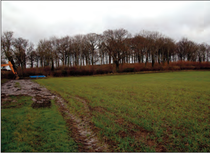
Plate 1 The site of the access track on the north side of Field 2
