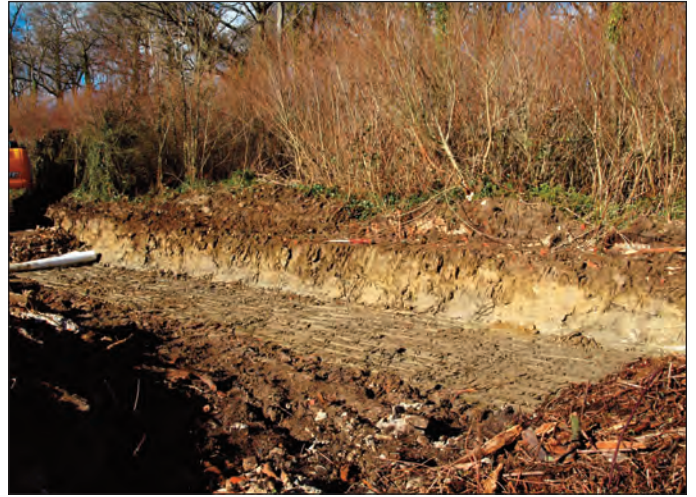
Plate 8 Oblique section view of access roadway on the east side of Field 2, looking north-west, 1m scale
