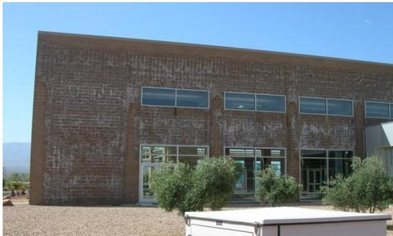
Do not get fooled that the moisture will only travel to the outside of the building. The interior adjacent rooms are typically maintained at 75°F and say 40% RH. This condition has a grain / lb content of 51.8 so the moist air in the pool room will travel to the other interior rooms. All pool room partitions need a vapor barrier. All windows and doors need to have a very tight seal to prevent moisture migration.
