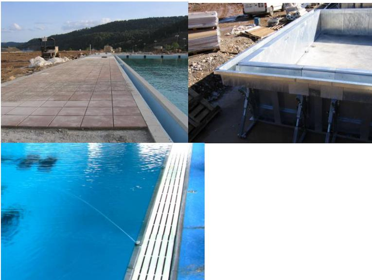
Both skimmers and gutters take surface water from the pool and get it to the filter system by piping. The larger pools usually have gutters. There are many types of gutters – some get the water off the surface more effective and efficiently than others – but their primary function is the same. Get the water to the filters.
