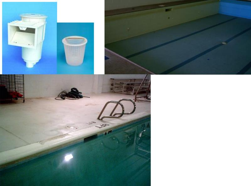
It can also be accomplished by a trough along the outer top edge of the pool around the total perimeter. These are called gutters.
