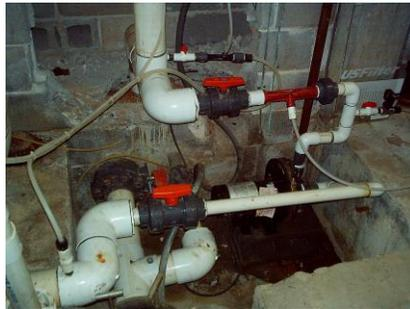
There are also smaller valves that can bleed air from filters and control the flow of chemicals into PVC lines. The same rules apply about handle direction as related to off/on.
