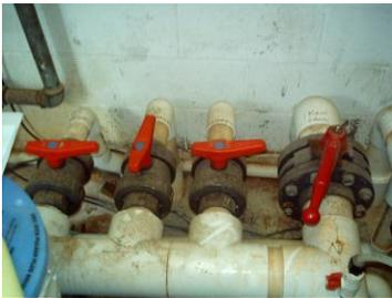
In this picture numbering the valves from left to right – the 1<sup>st</sup> and 3<sup>rd</sup> valve are closed – the second valve is open – the 4<sup>th</sup> (larger valve) is 90% open.
