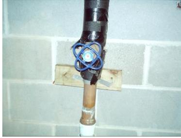
This usually turns the city (make up) fresh water supply off and on to fill the pool. Clockwise rotation of the handle closes the valve – counterclockwise rotation opens the valve and turns on the water. This is how the pool water level is controlled. Pool water level can be critical to proper operation of pool equipment.
