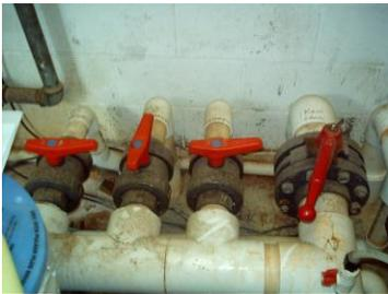
In this picture numbering the valves from left to right – the 1<sup>st</sup> and 3<sup>rd</sup> valve are closed – the second valve is open – the 4<sup>th</sup> (larger valve) is 90% open.
