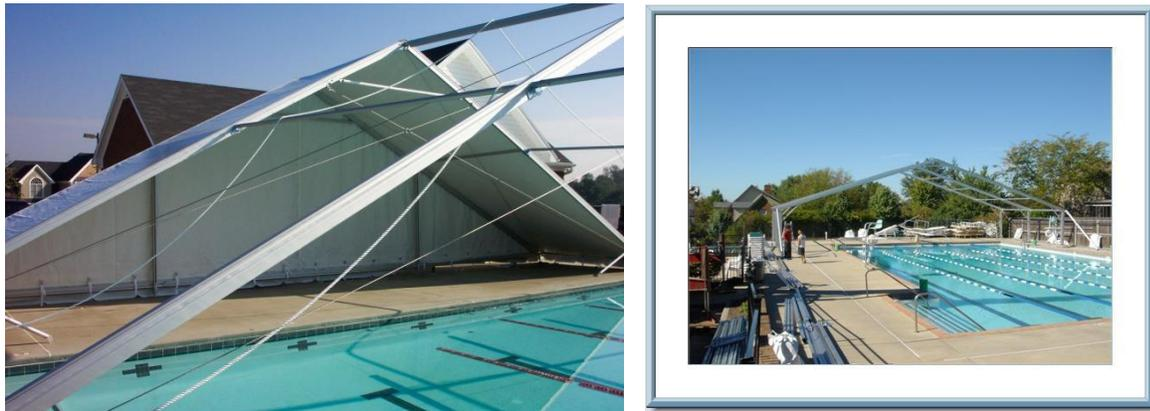
The aluminum beams are bolted together and lifted into place.
