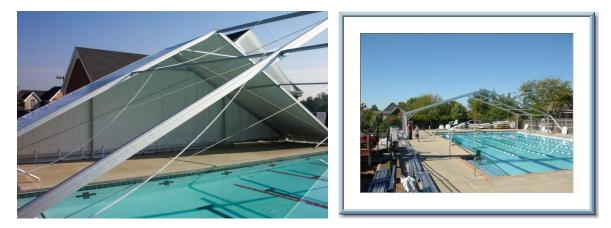
The aluminum beams are bolted together and lifted into place.
