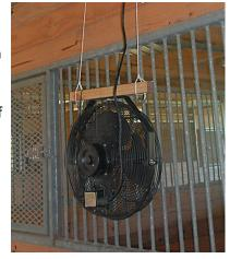
to shut off the fan. Check the overhead temperatures with a large thermometer by hanging it where you plan to put the fan or by putting the thermometer on a (non-conductive) pole and holding it up where the fan is to go.
