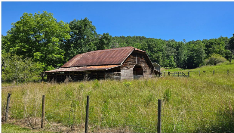
Driving 112328 Barn Rusty Roof
