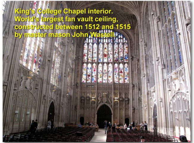
Fan vault is a Gothic style vaulted ceiling in which the ribs are all of the same curve and spaced equidistantly, in a manner resembling a fan.
