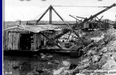
Digging with Dredges
