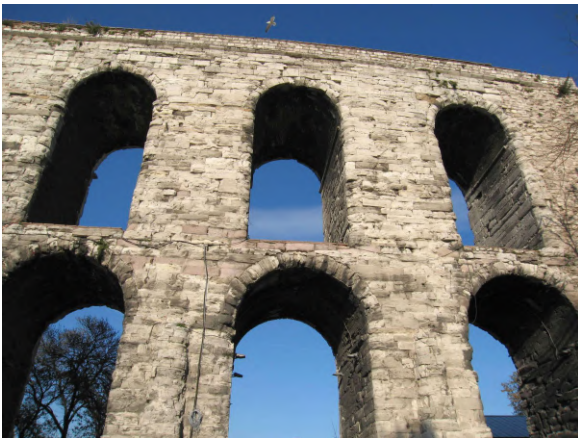
Valens Aqueduct IMG_9397 Roman 368 AD
