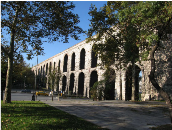
Valens Aqueduct IMG_9387 Roman 368 AD
