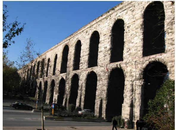
Valens Aqueduct IMG_9389 Roman 368 AD
