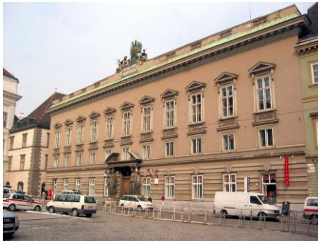
Palais Pallavicini #4169 Built 1784
