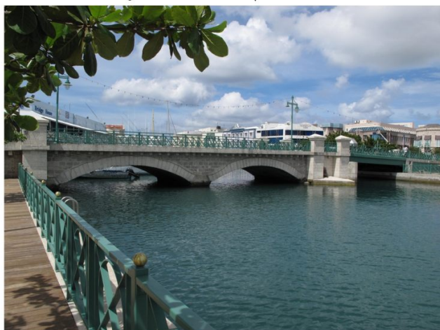
Bridgetown #0169 Chamberlain Bridge
