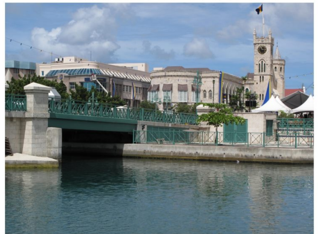
Bridgetown #0168 Chamberlain Bridge
