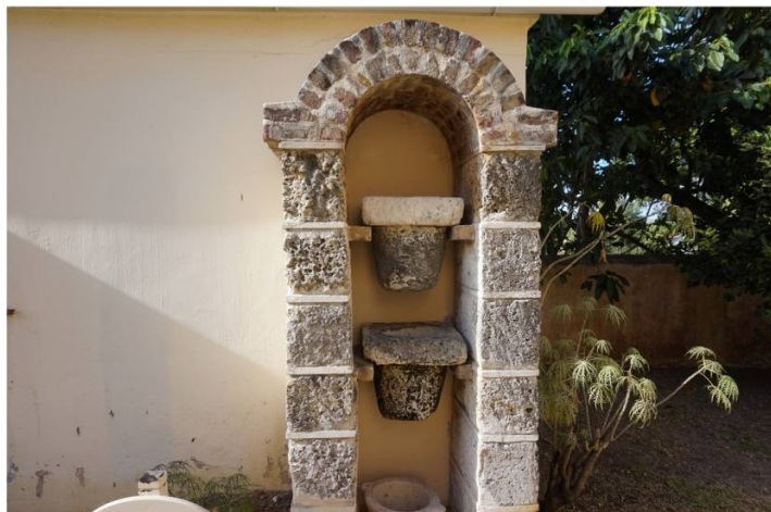
George Washington House #2763 Drip Water Filtration
