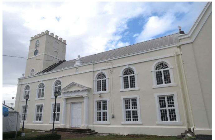
Speightstown #3545 St Peter's Church 1837 Rebuilt After Fire 1980
