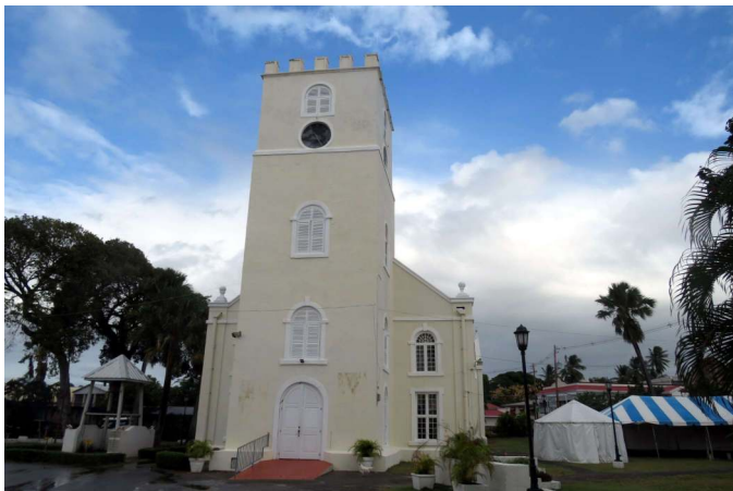
Speightstown #3544 St Peter's Church 1837 Rebuilt After Fire 1980
