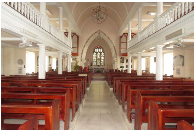
Speightstown #3547 St Peter's Church 1837 Rebuilt After Fire 1980
