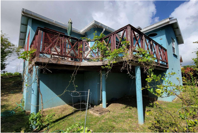
St Philip #0004 Rear of House
