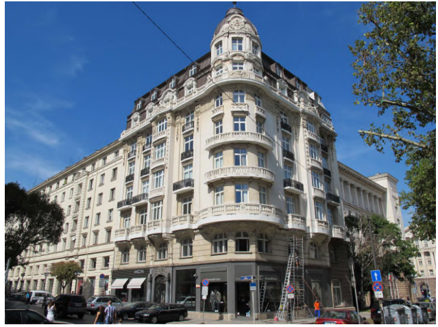
Misc #8019 Interesting Old Building
