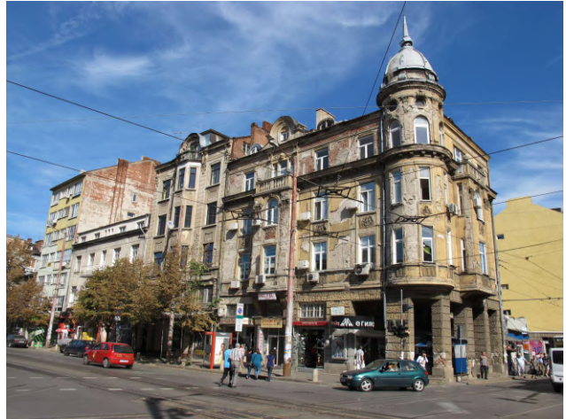
Misc #8221 Interesting Old Building
