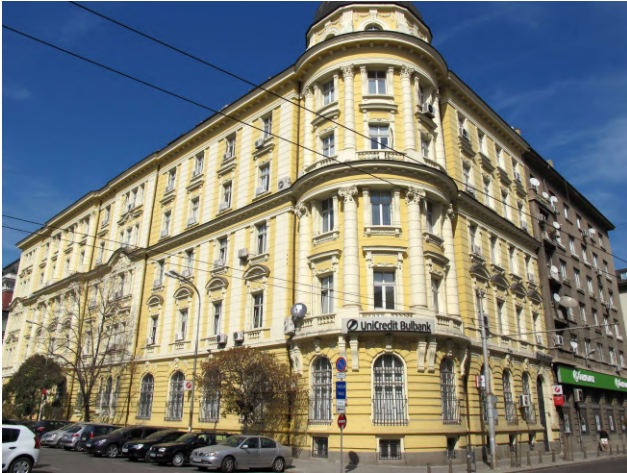
Misc #8039 Interesting Old Building
