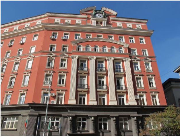
Misc #8018 Interesting Old Building
