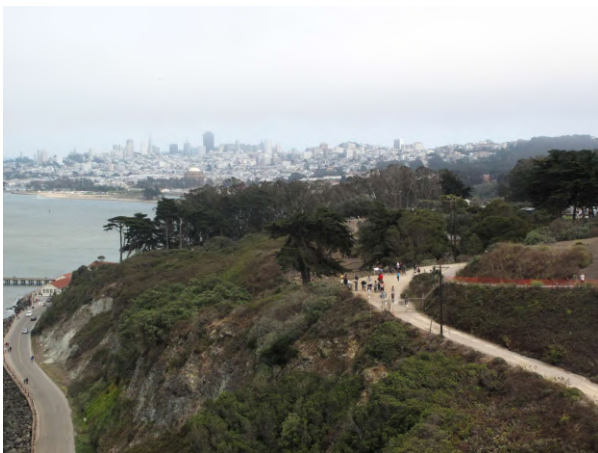
Golden Gate Bridge #1794
