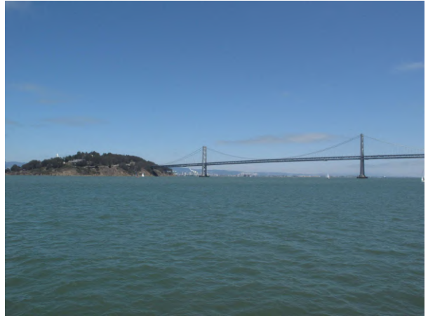
Ferry Sausalito to San Francisco #1016 Bay Bridge
