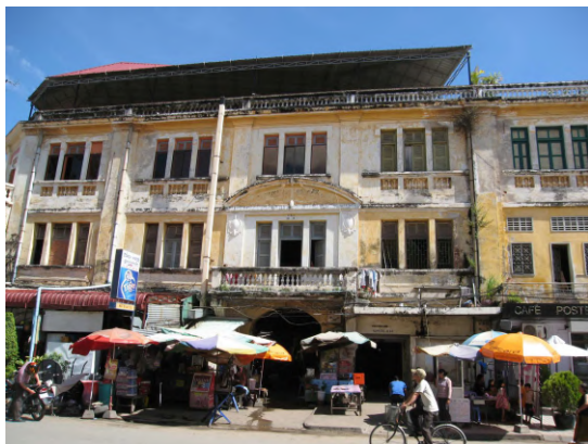
IMG_9408 French Colonial Building
