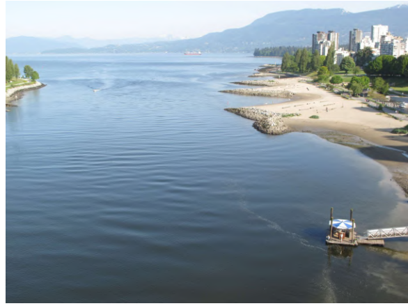
Burrard St Bridge #4440
