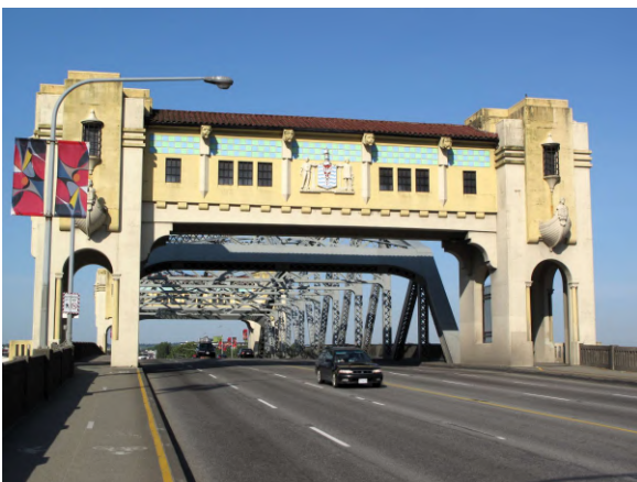
Burrard St Bridge #4435
