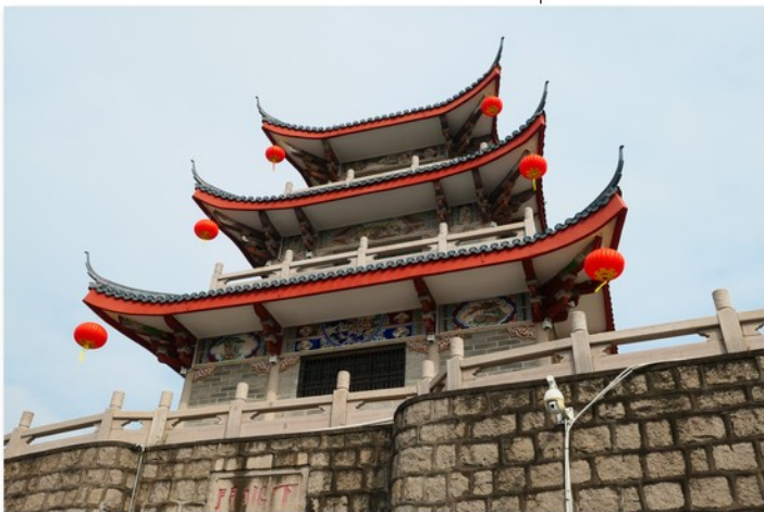
P1281596 Lower Water (Xiashui) Gate & Ruins of Ming City Wall
