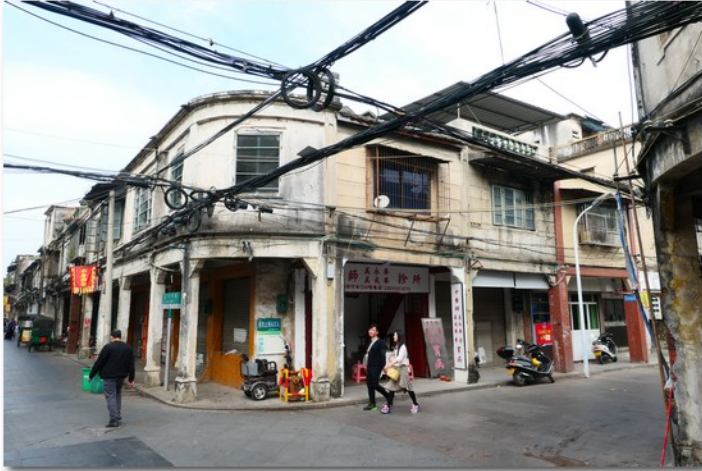
P1281867 Old Neighbourhood Electric Wires
